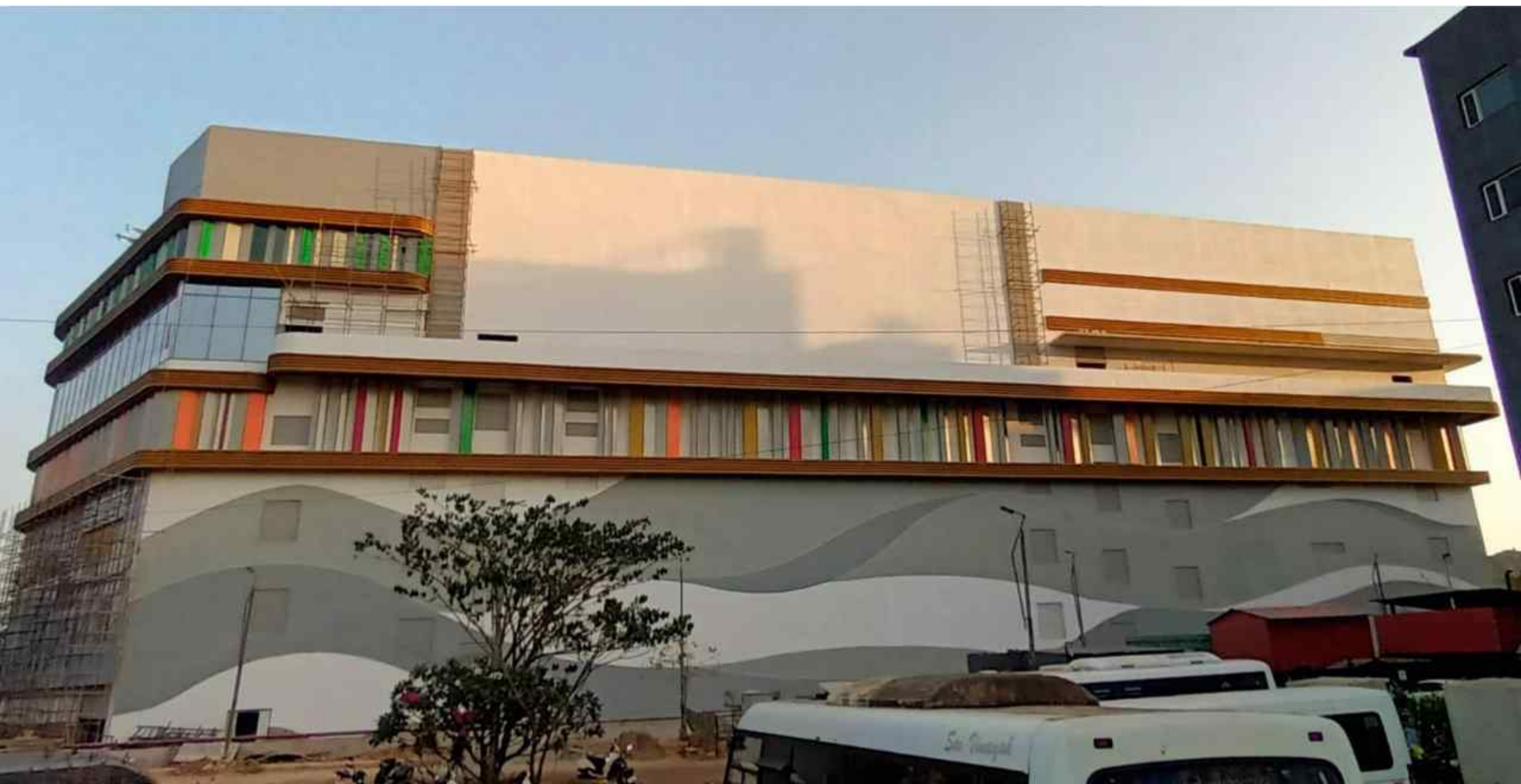
North side elevation of the building
