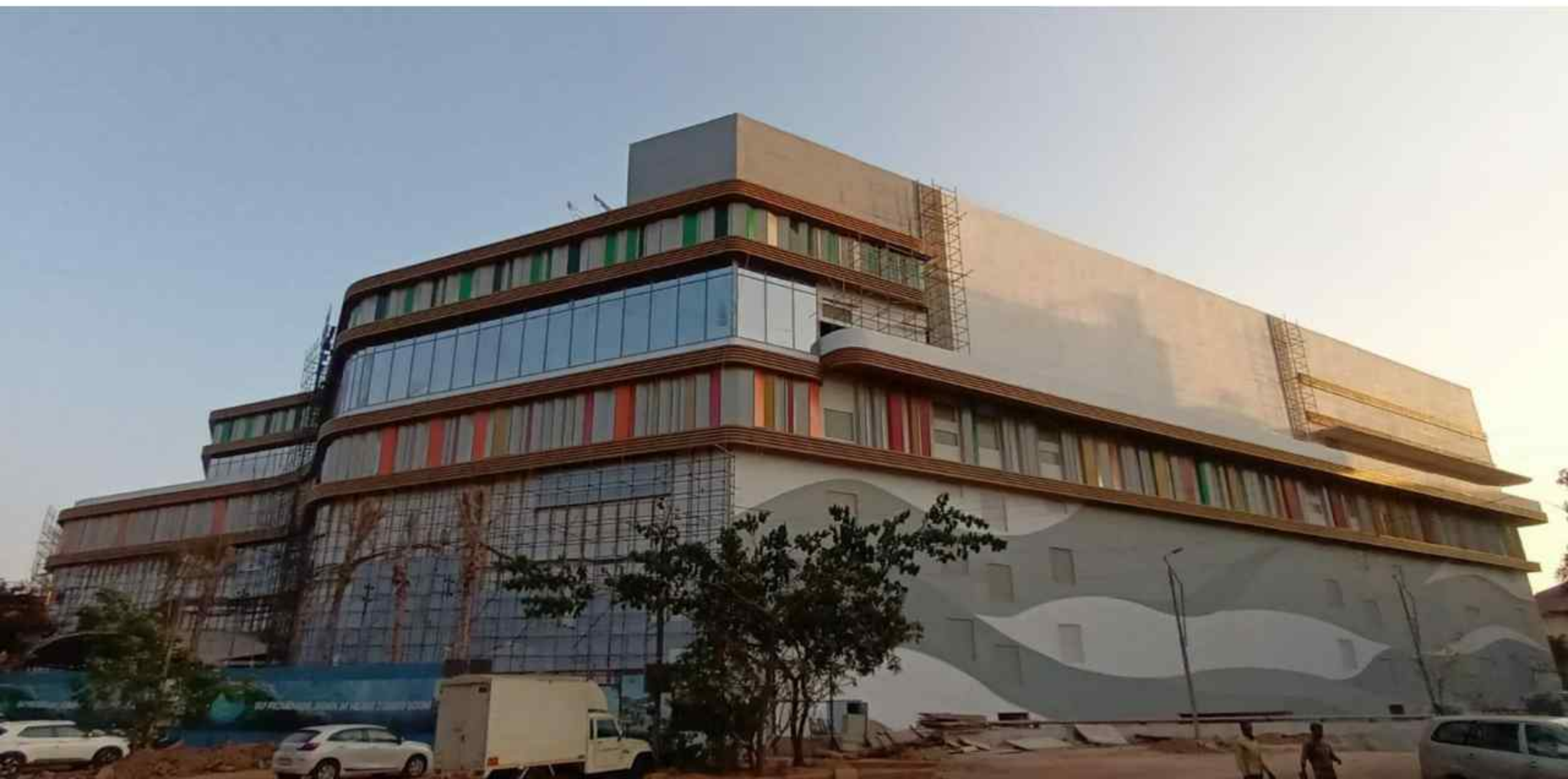
North east Corner view of the building
