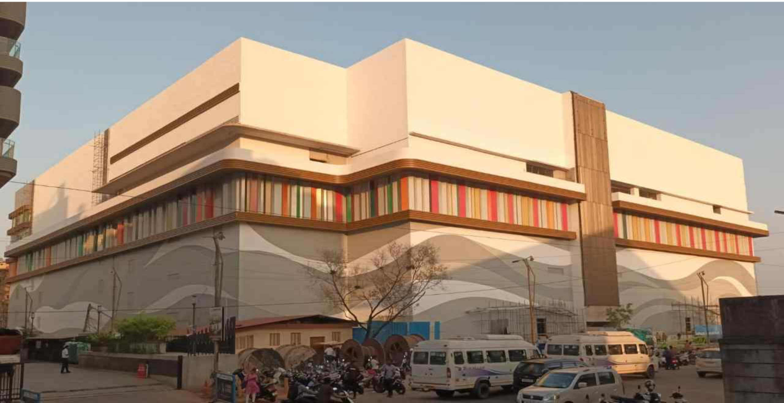
North west Corner view of the building
